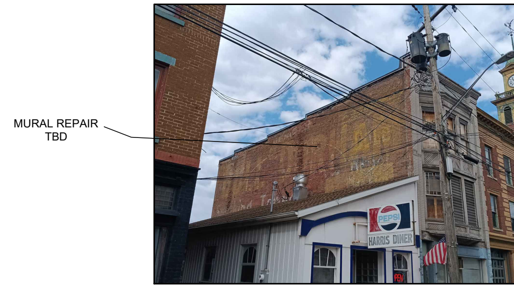
SIDE (SOUTH) FACADE
