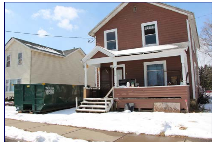
Homes in the Flats neighborhood impacted by Tropical Storm Lee
