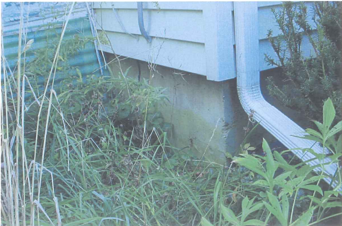
Photo 3. Poured concrete foundation at the northeast corner of 130 Southside Drive.
