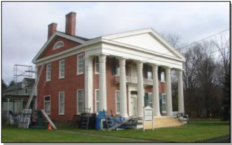
Historic building renovations are currently underway in the Village of Nichols.
